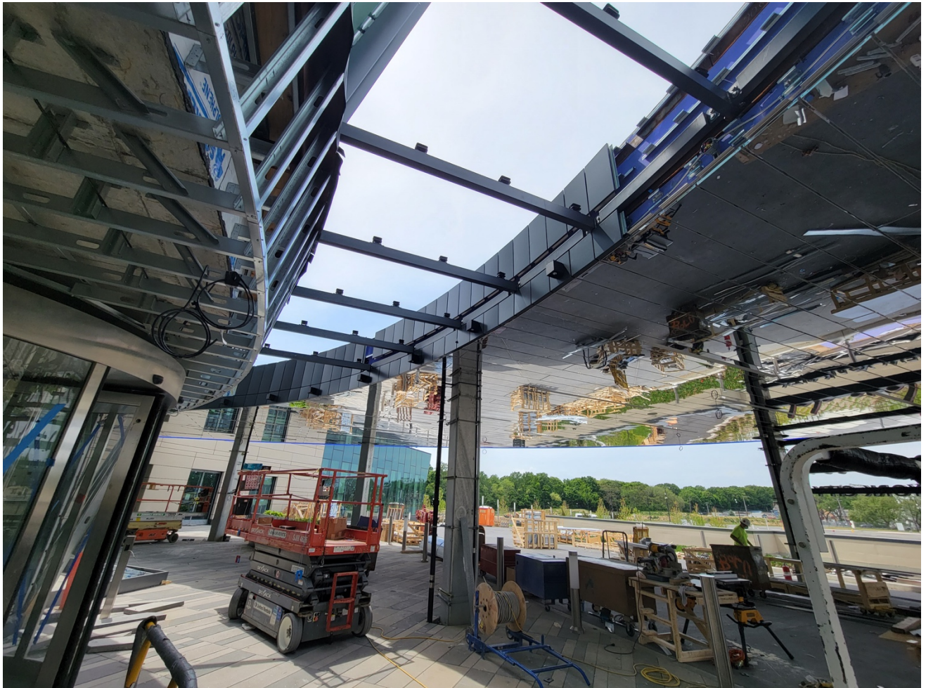
Main Entrance Resorts World Casino Canopy
