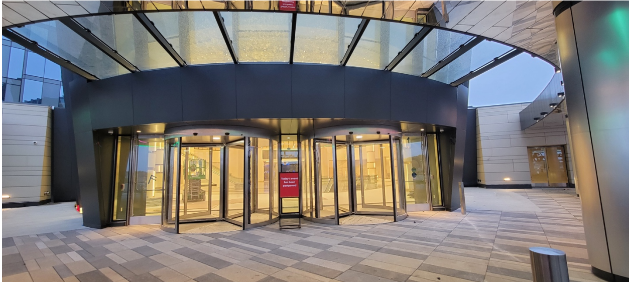
Revolving Glass Doors Entrance Finished Work
