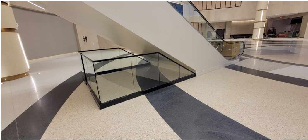
Finished Work Glass Handrails/Lobby Resorts World Casino
