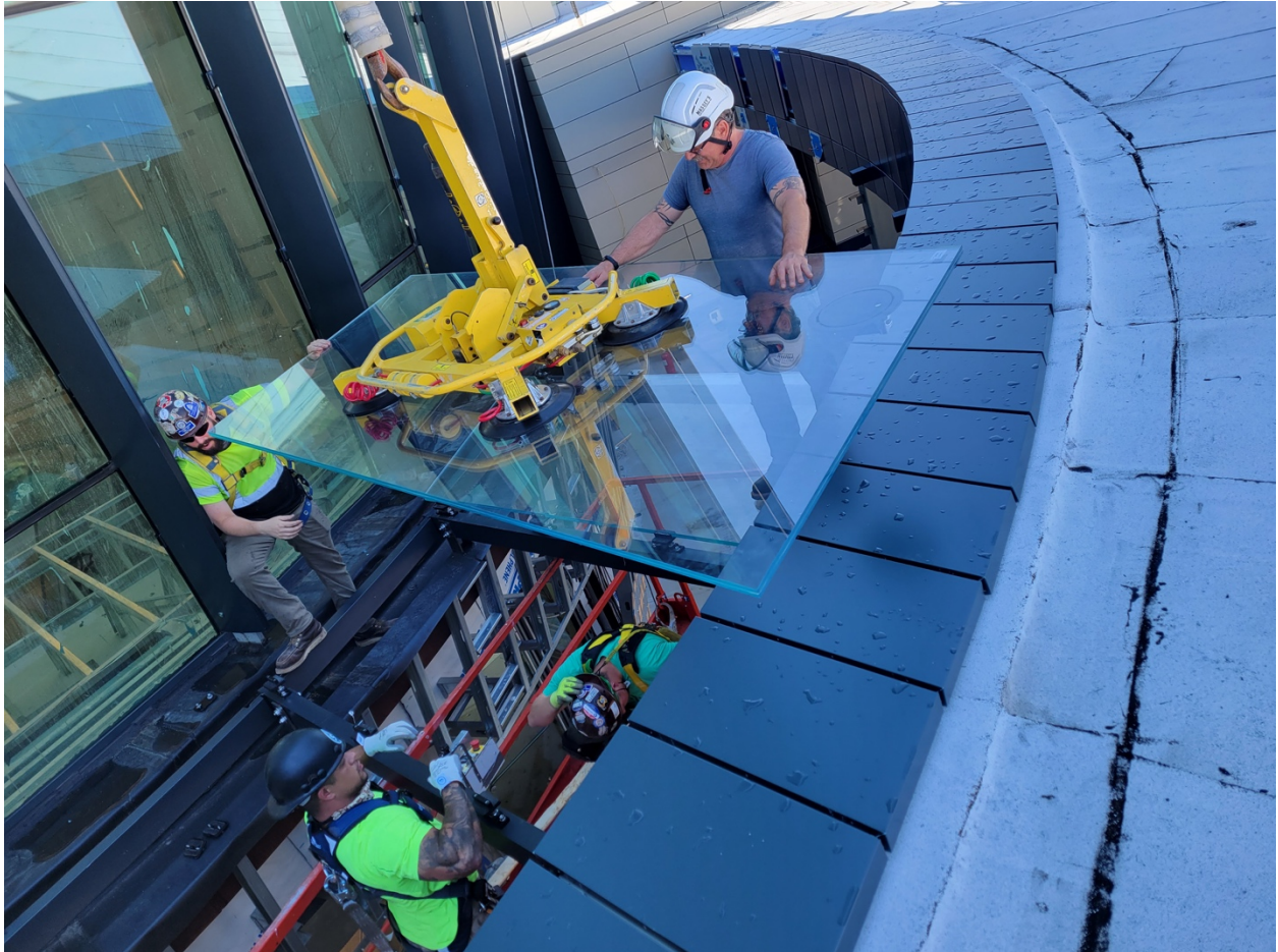
Installation Glass Roof/Canopy Main Entrance
