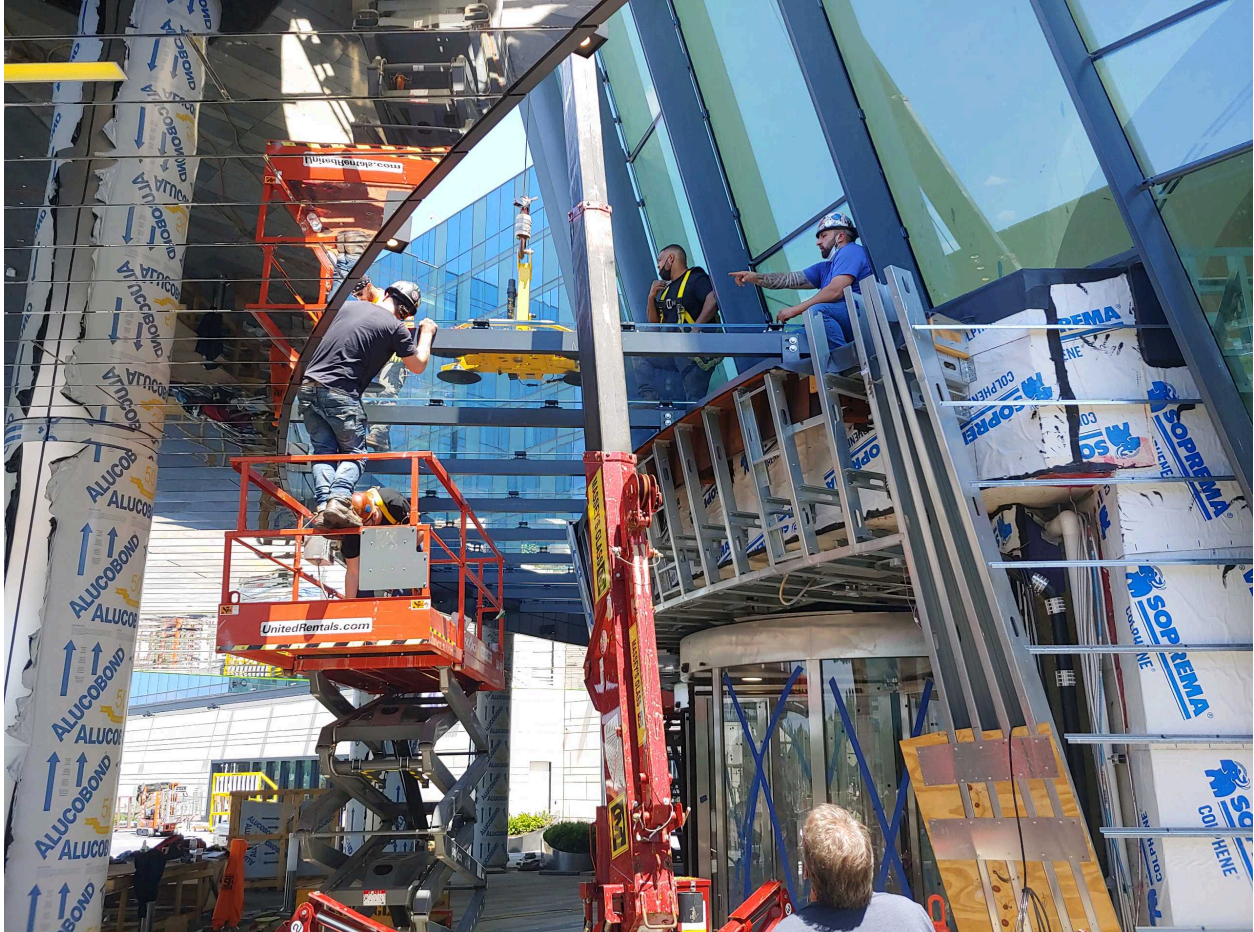
Installation Glass Roof/Canopy Main Entrance
