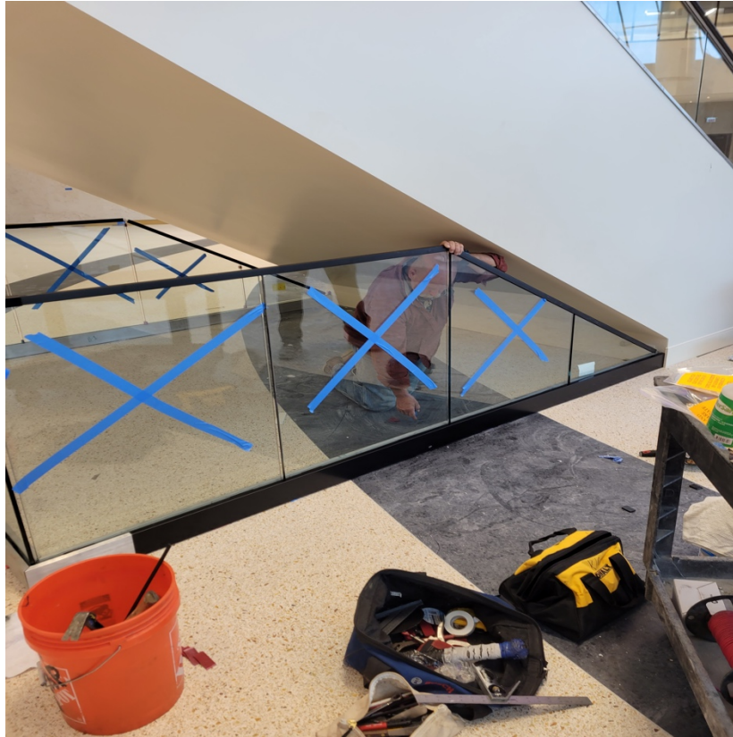
Glass Handrails/Staircase Resorts World Casino
